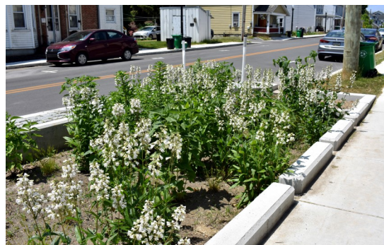
Rain Garden Along B Street
